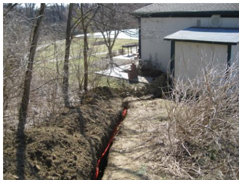
Increased Electric Service to 200 Amps
