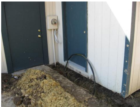
Increased Electric Service to 200 Amps
